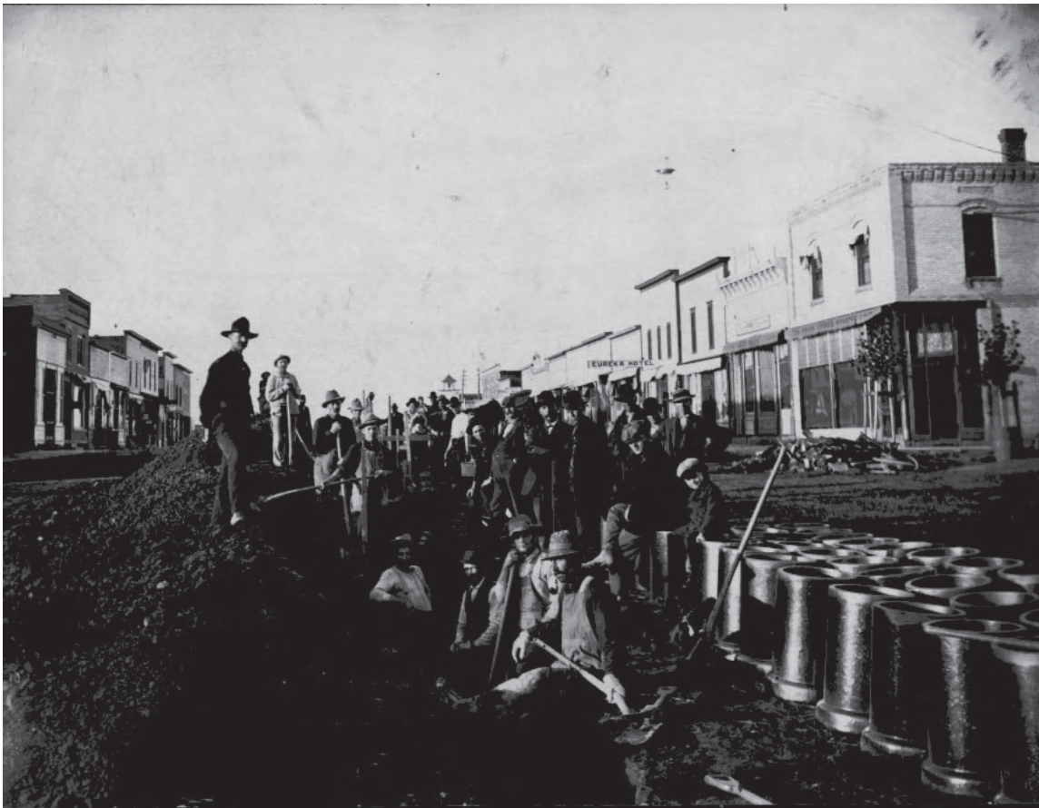
Laying sewer pipes on Avon's Main Street. The corner building was built about 1907 and is still being used for a grocery store--Ron's Market.
